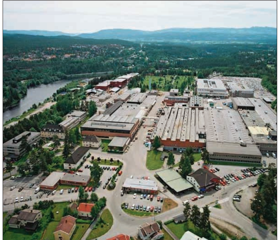
Dresser-Rand's facility in Kongsberg, Norway
