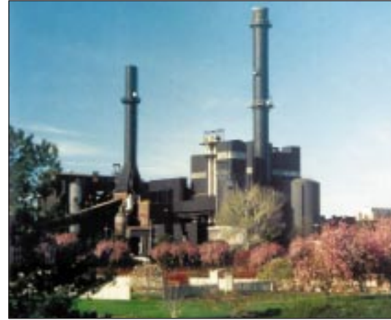
The power generation facility at Iowa State University, in Ames, Iowa, produces electricity for the campus, as well as heating and air-conditioning through steam extraction.
